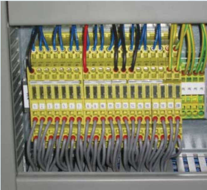
6 mm wide surge protective modular terminal block, 2-pole, with cage clamp connection. Earthing via DIN rail or terminal.
