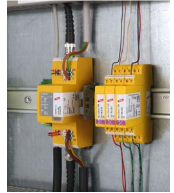
Space-saving and application-optimised 3in1 arrester DEHNvario
